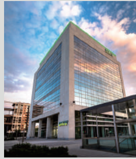
HQ Mansion of DKV, Spain
